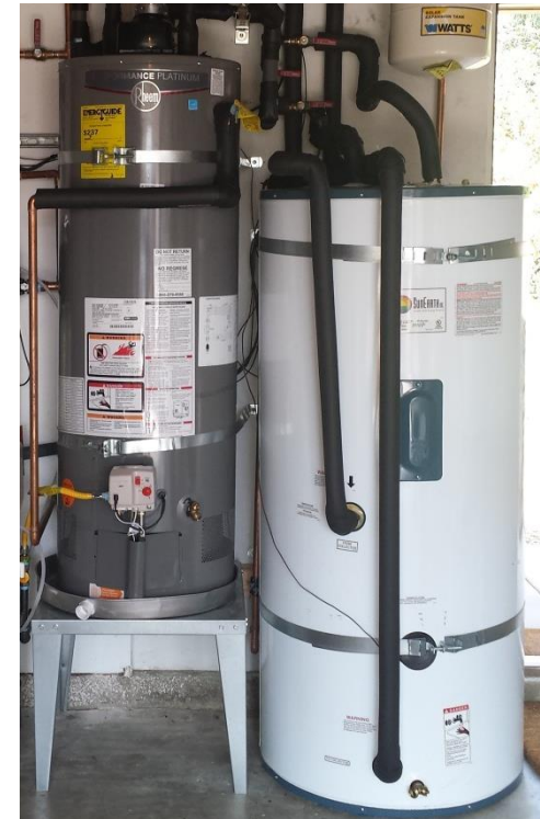
Solar storage tank next to existing water heater
