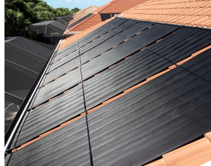
Unglazed Collectors (Generally for Pool Heating)
