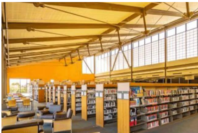
The public library is one of five buildings supported by the Energy Roadmap in Cupertino.
