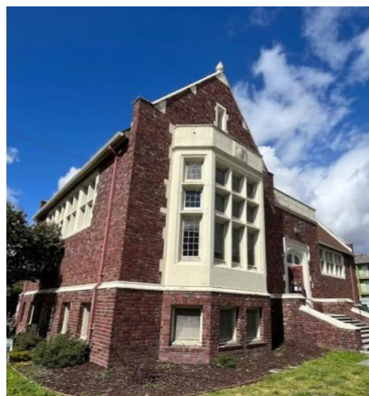
The Temescal Branch Library in Oakland, CA.
