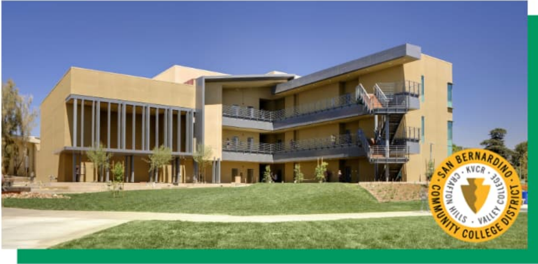
SBCCD is upgrading the interior lighting at San Bernardino Valley College North Hall and Library
